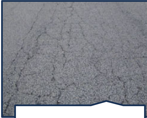
Alligator Cracking
