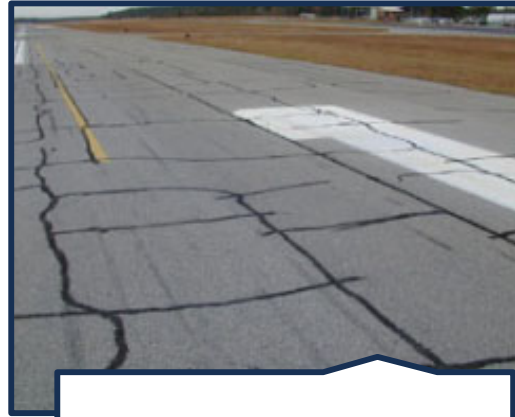
Block Cracking
